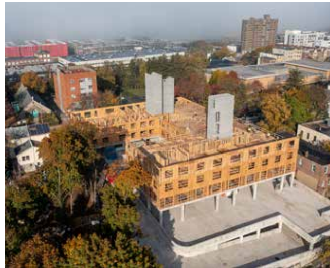
Summit on Hudson mid-construction
